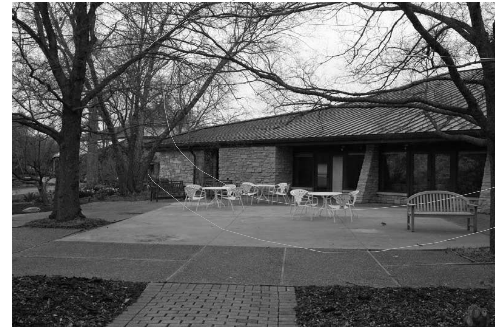
EXTG LUSSIER TERRACE ZONE TO BE REPLACED.
