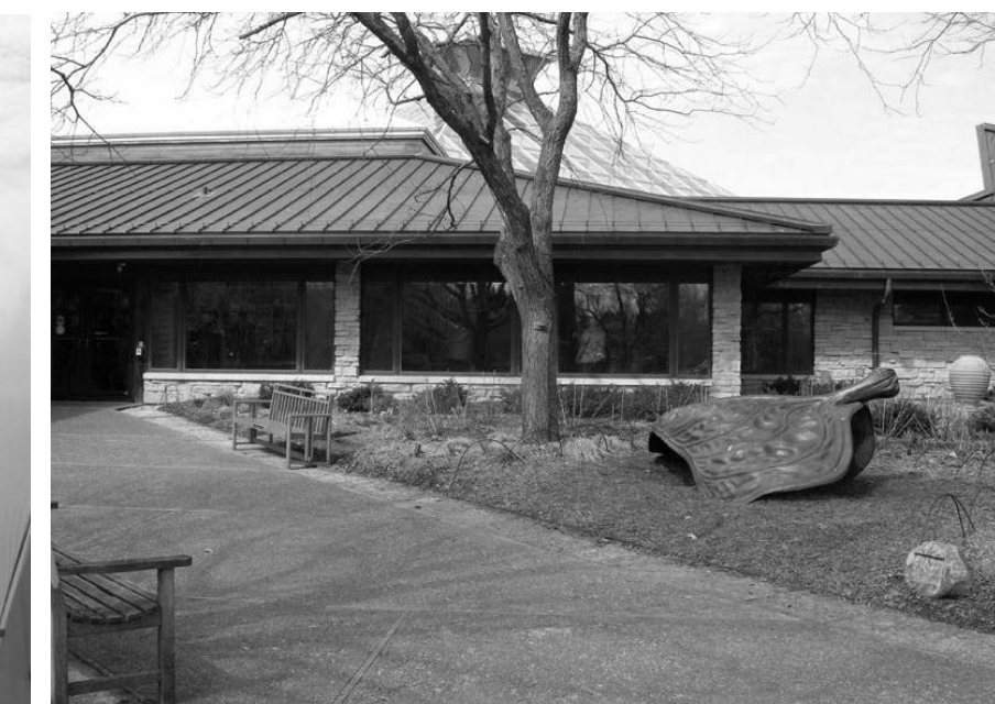
EXTG LOBBY EAST ELEVATION
